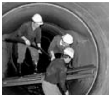
污水管線施工
