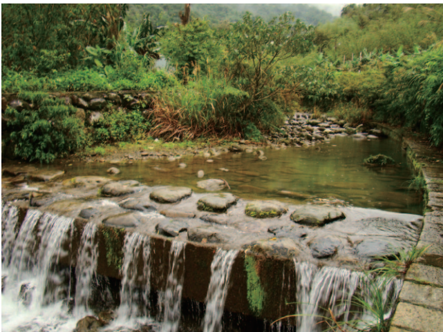
阿柔坑溪透過「生態工法」，不僅達到穩定河床的功能，也回復當地多元生態。 The project used ecological engineering techniques to stabilize the Aroukeng River riverbed and restore the area's diverse ecology.
